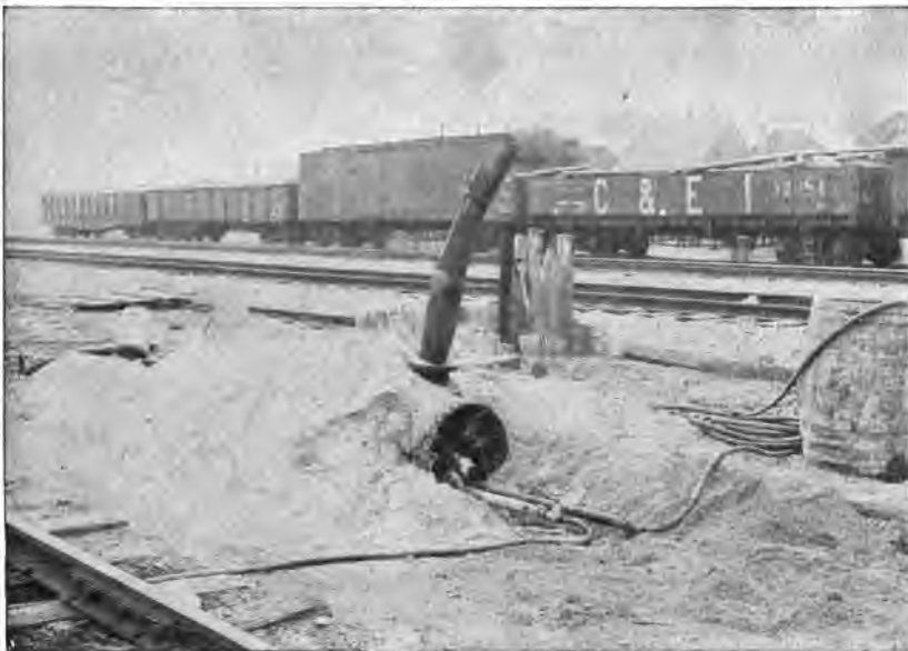
FIG. 4.—METHOD OF HEATING SAND.
